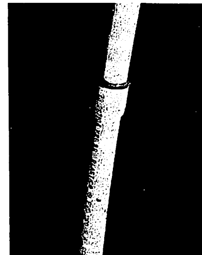
4. Assemble 25 ft. lengths of ¾" schedule 40 PVC pipes by gluing a 20 ft. length to a 5 ft. length. Thinner grades of PVC pipes are not recommended since they may crease immediately above the ground level.
